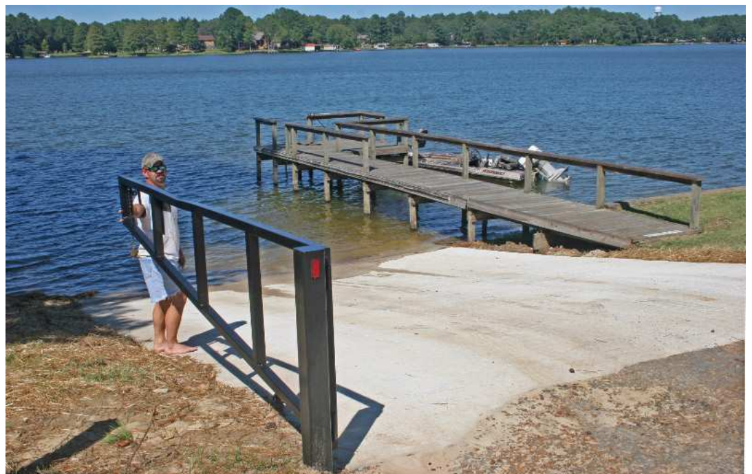
The new boat ramp, with just enough water to float in...
