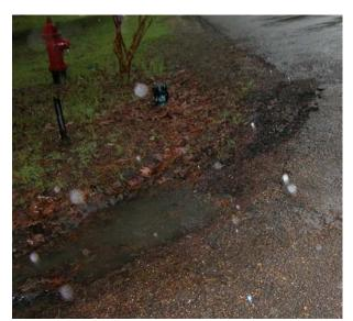
Almost all roads within our system at one time had draining ditches on the sides to manage the flow of the water off the roads. Over the years these have filled up. The dirt dauber feels this issue needs to be addressed before road overlays are taken to extend the life of the road being worked on and to divert the water properly.
